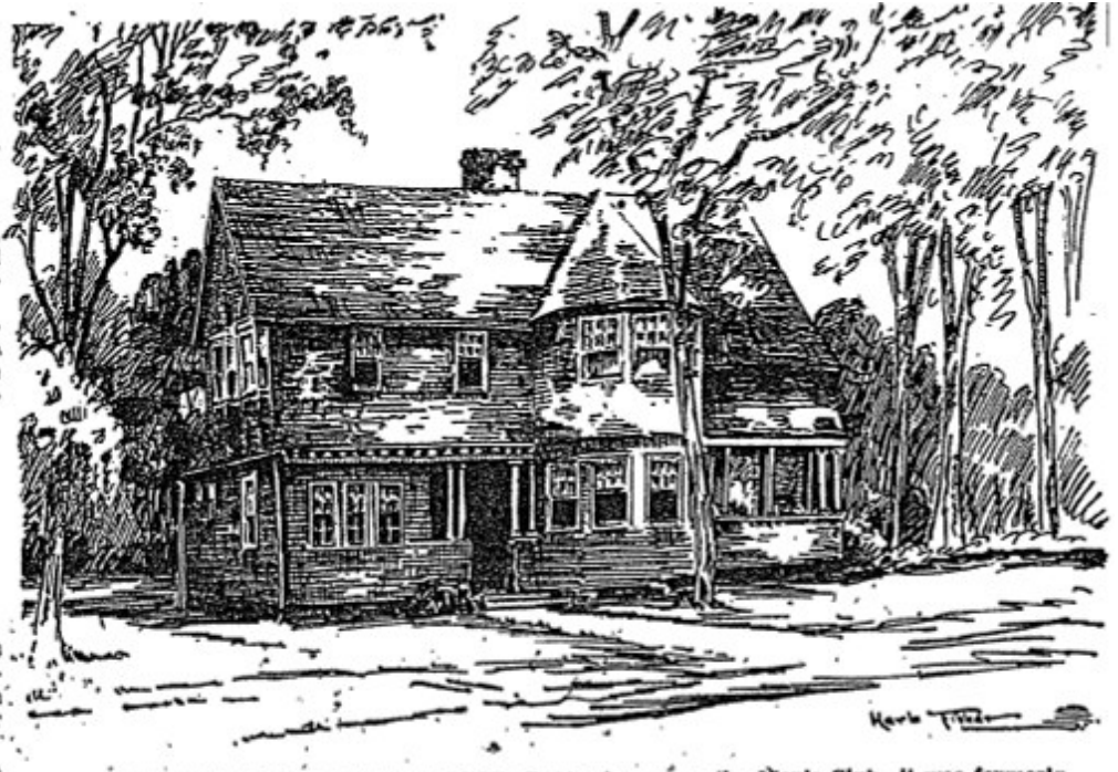
THE GLEN RIDGE CLUB HOUSE. Better known as the Men's Club it was formerly opened in 1885. It became the social center of the community. In 1933 the club was given up and the house demolished. It occupied the site of the present post office.
