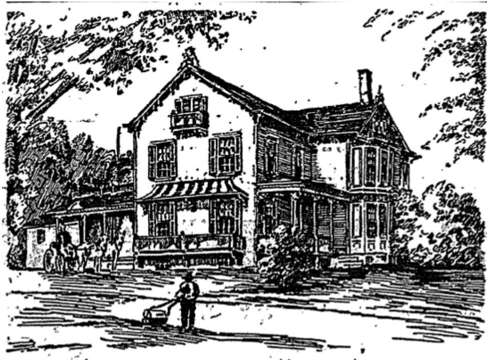
RESIDENCE OF JARVIS PELOUBET. Located on Lincoln avenue, a short distance west of Clinton street, this house is still standing. Most of the gingerbread has been taken off, but the lines of the house remain the same.
