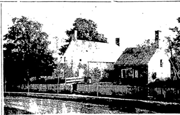
IN THE OLD DAYS this famous Bloomfield home, the Thomas Cadmus house at Washington and Clinton streets, had slave quarters behind the main building. The Cadmus house, now owned by Dr. Melvin D. Greer, is shown as it appeared years ago.
