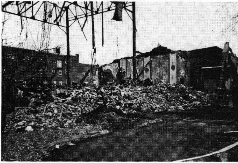
The demolition of the Royal Theatre.
